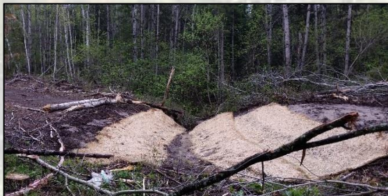
Winter crossing removal with straw mats
